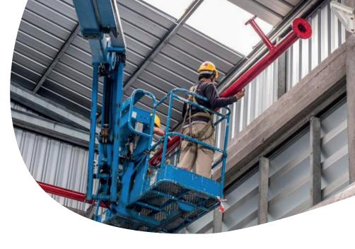
worldwide each year. They consist in a water supply system, providing adequate pressure and flowrate to a water distribution piping circuit, onto which fire sprinklers are connected. This network of distribution pipes is the essential component of a sprinkler system.
